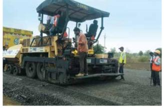
Dry Lean Concreting commencement in Nagpur Ring Road by using concrete batching plant having capacity of 120 cum per hour
