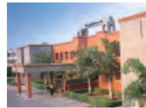
Noida Central Plant
