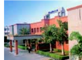
Noida Central Plant
