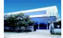
Subros Tool Engineering Centre
