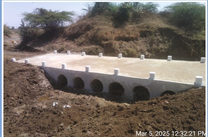
Construction of Culvert at village Harsani
