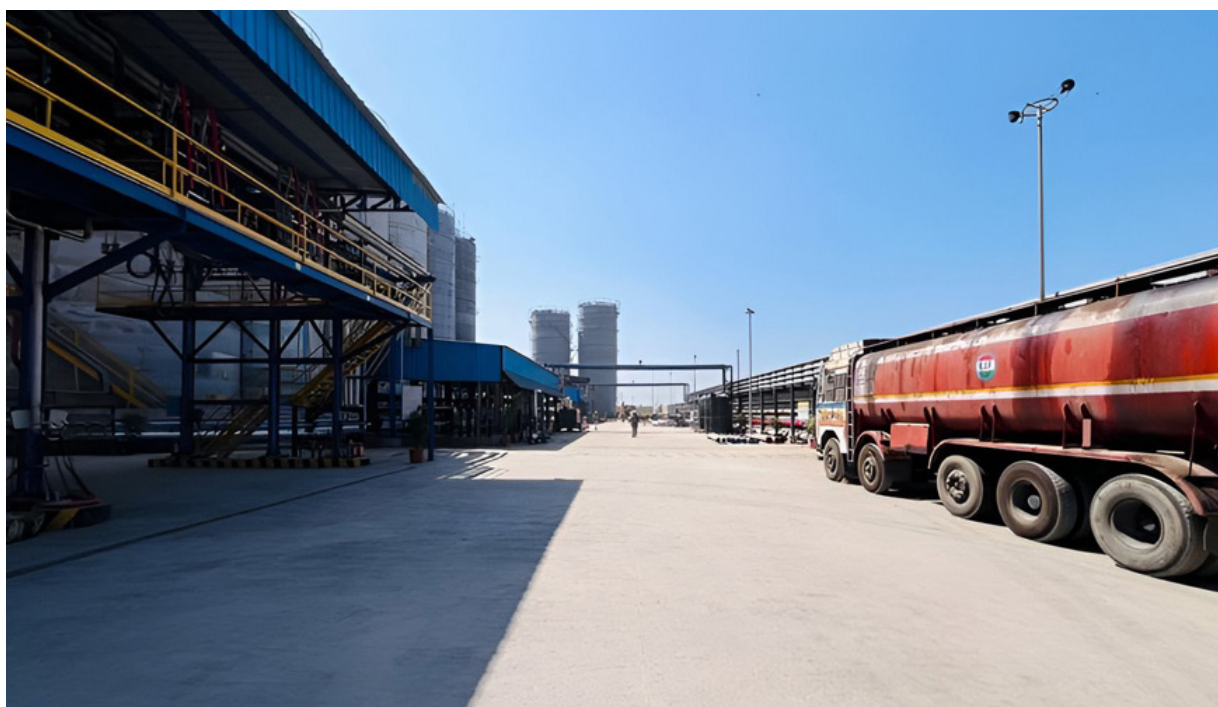
New liquids terminal at JNPT
