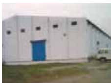
Pant Nagar Plant Omax Autos Limited Vill.& P.O. Lalpur, Rudrpur-Kichha Road, Khasra No.180A, 181,183,175 Distt.U.S.Nagar Uttrakand-263153
