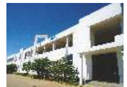
Bangalore Plant Plot No.-6, Bomassandra-Jigani Link Road, Bomassandra, Bangalore, Karnataka - 560099
