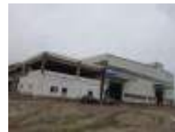
New Railway Plant: Village Kandhawan, Maharajganj, Raebareli, Uttar Pradesh, 229404
