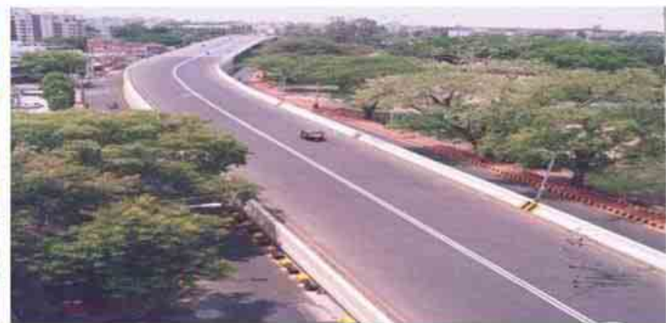
Project: Nagpur Flyover
