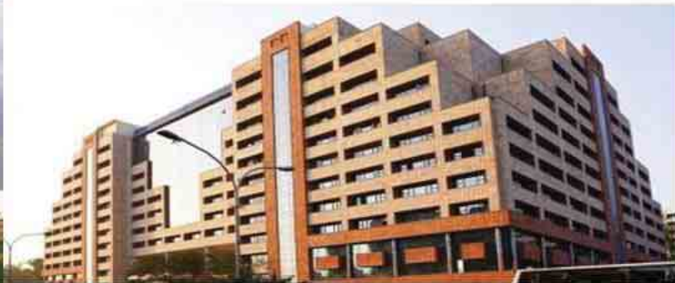
Project: Cabinet Secretariat Building, New Delhi
