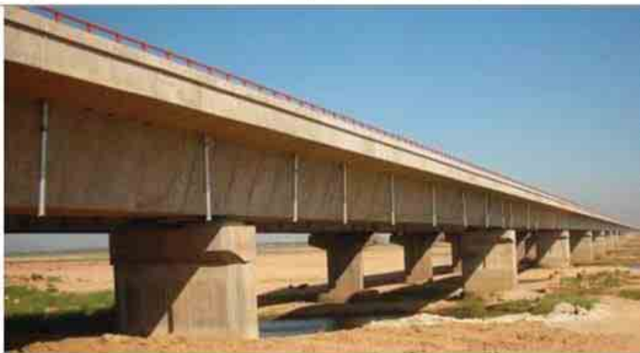
Project: Bridge on River Sone (Longest bridge of GQ)
