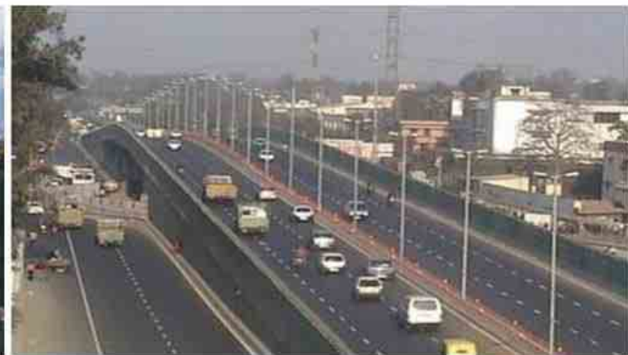
Project: Britania Flyover at Ring Road, Lawrence Road, Delhi
