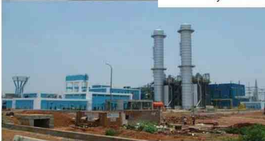
Project: Gowtami Powr Project, Peddapuram Scope: 460 mw combined cycle power plant at Kakinada
