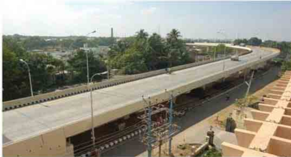
Project: Kovilpatti Flyover, Chennai
