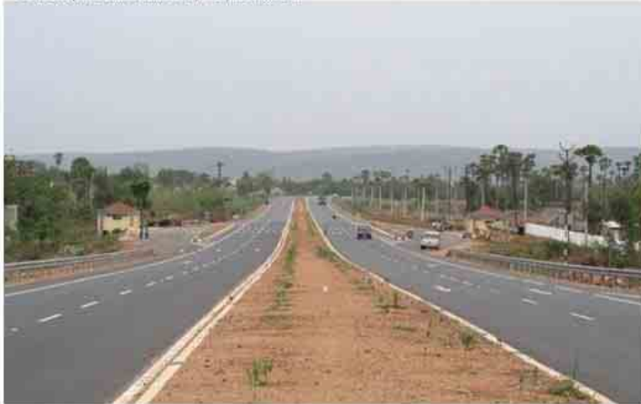
Project: AP-Package between Vishakapatnam and Champavati river of NH-5 for NHAI JV with Unitech Ltd., New Delhi
