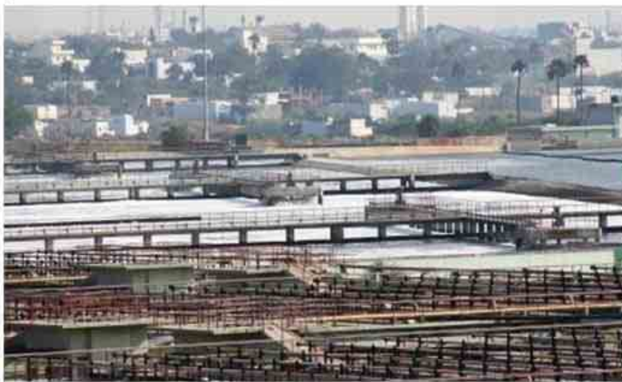
India Biggest water treatment plant, Amberpet, Hyderabad
