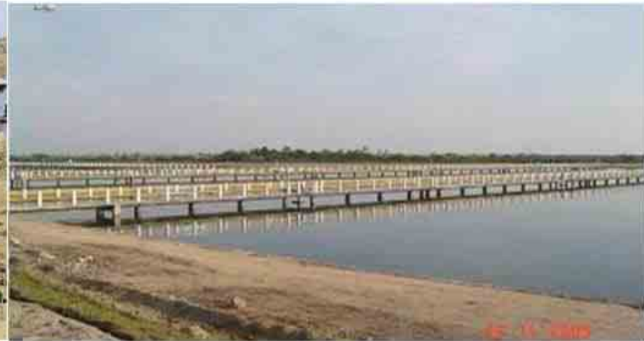
Project: UGD Scheme, Bellary - Karnataka Scope: 15 MLD & 30 MLD sewage treatment plant, SWG/RCC pipelines.
