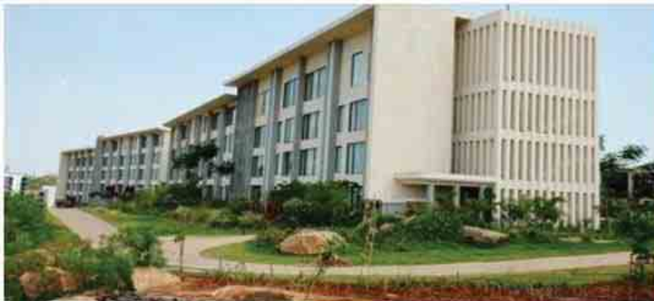
Project: ISTA Hotel, Hyderabad Scope: 5 Star Hotel & Swimming Pool
