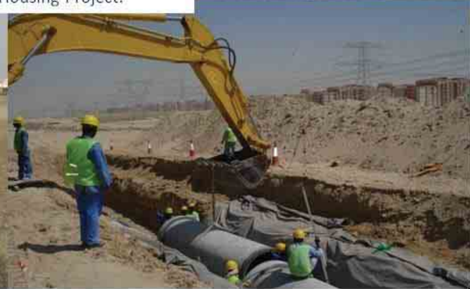
DEWA Pipe Line Project, Dubai, Package- 512A
