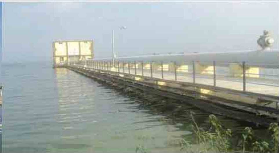
JACK WELL CUM PUMP HOUSE - MIHAN
