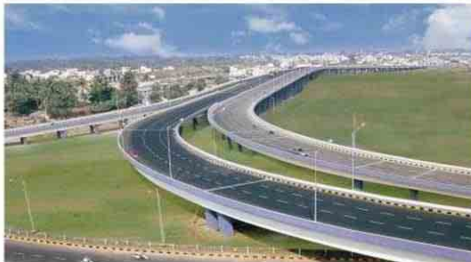
Project: Bangalore Elevated Flyover
