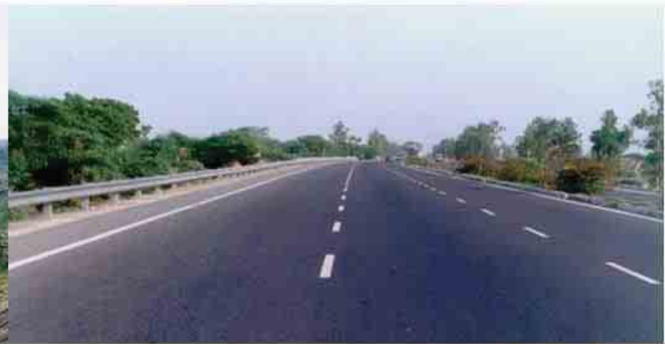
Project: NHAI-Six Laning of NH-1 for 15 Kms. of Delhi Border to Samalkha section in Haryana state.
