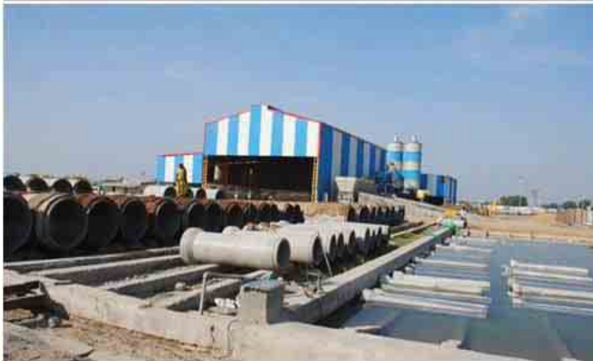
RCC PIPE MANUFACTURING UNIT- INDORE
