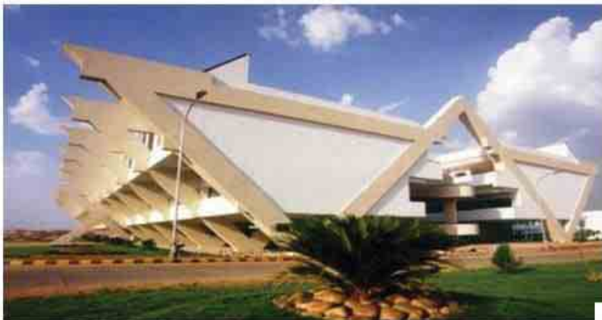
Project: NAC, Hyderabad (Reward received for early completion) Scope: Building, Infrastructure & ancillary structure..
