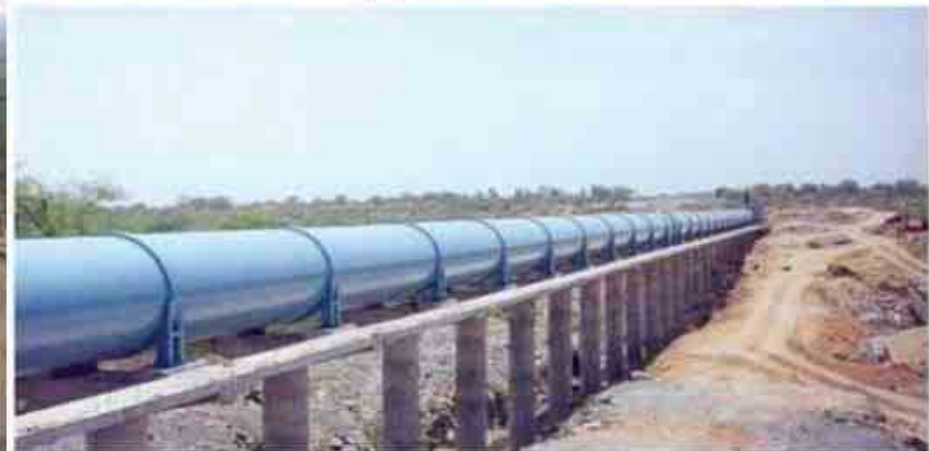
Project: Krishna Drinking Water Supply Project-Phase I
