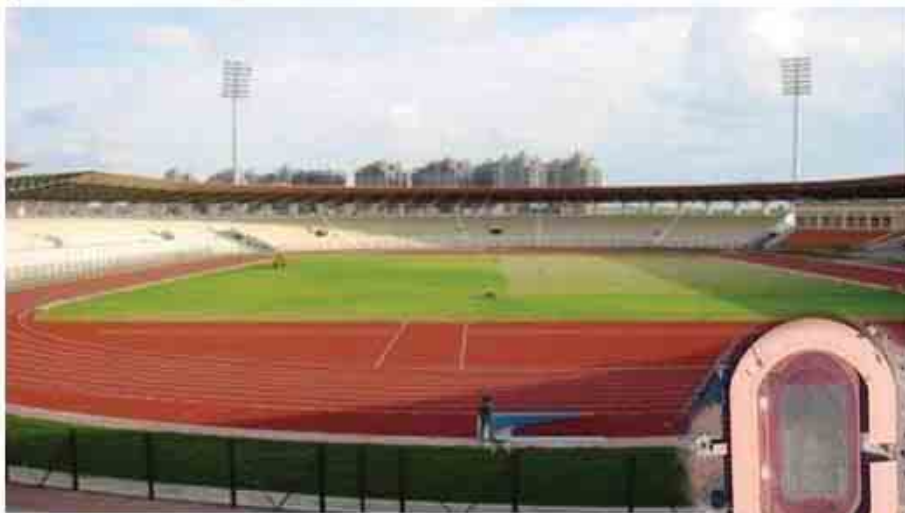
Project: GMC Balayogi Stadium, Gachibowli, Hyderabad Scope: Construction of Athletic Stadium for National Games 2002
