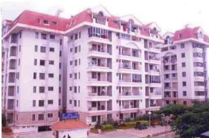
Project: SPPL White House, Karnataka.
