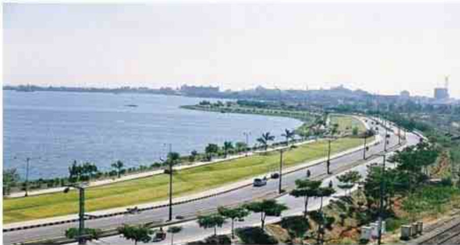
Project: Necklace Road under Buddha Purnima Project for Hyderabad Urban Development Authority, Hyderabad
