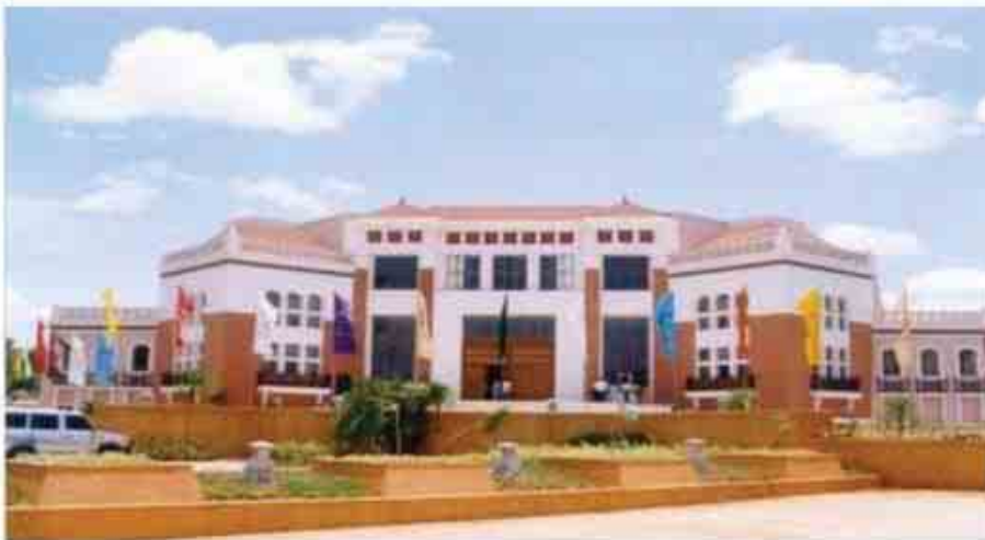
Project: Shilpakalavedika, Hyderabad Scope: Multistoried Build-Award received as outstanding structure - 2002
