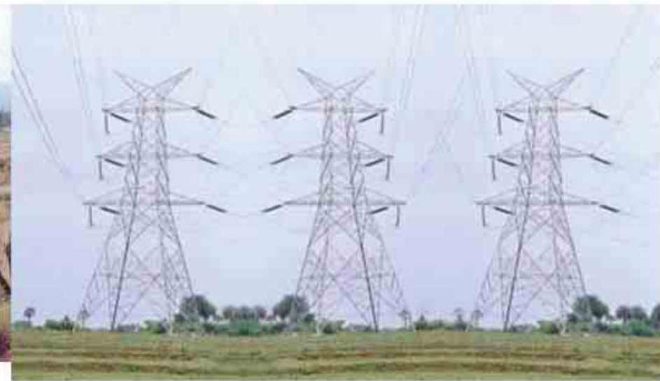
100 kms. Long 400 KV Transmission Lines, APTRANSCO, Khammam, AP. Completed in 13 months
