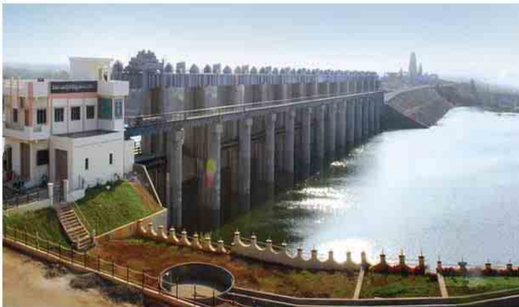
Project: Gundalkamma Reservoir Project, Ongole Scope: Water supply of 80,000 acres, Dam, bund, Right & Left canals
