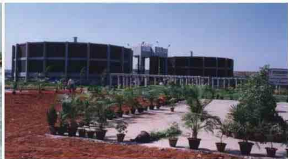
Project: V-Valley Scope: Civil works for 60 MLD waste water treatment plant
