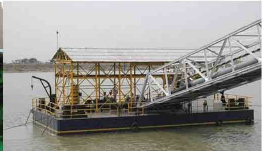
FLOATING BARGE - NADIA, WEST BENGAL
