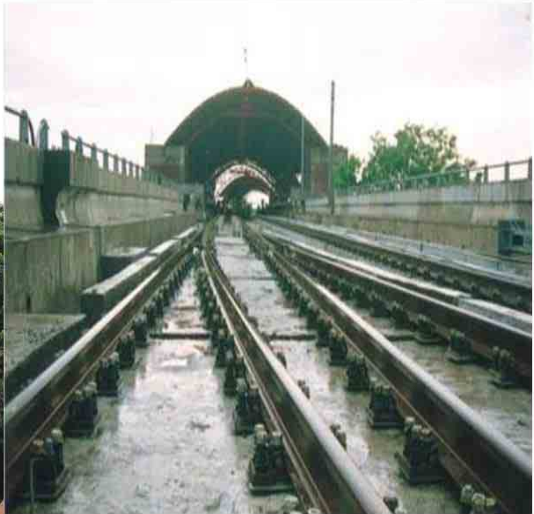
Project: Delhi Metro Rail Corporation Limited - Delhi
