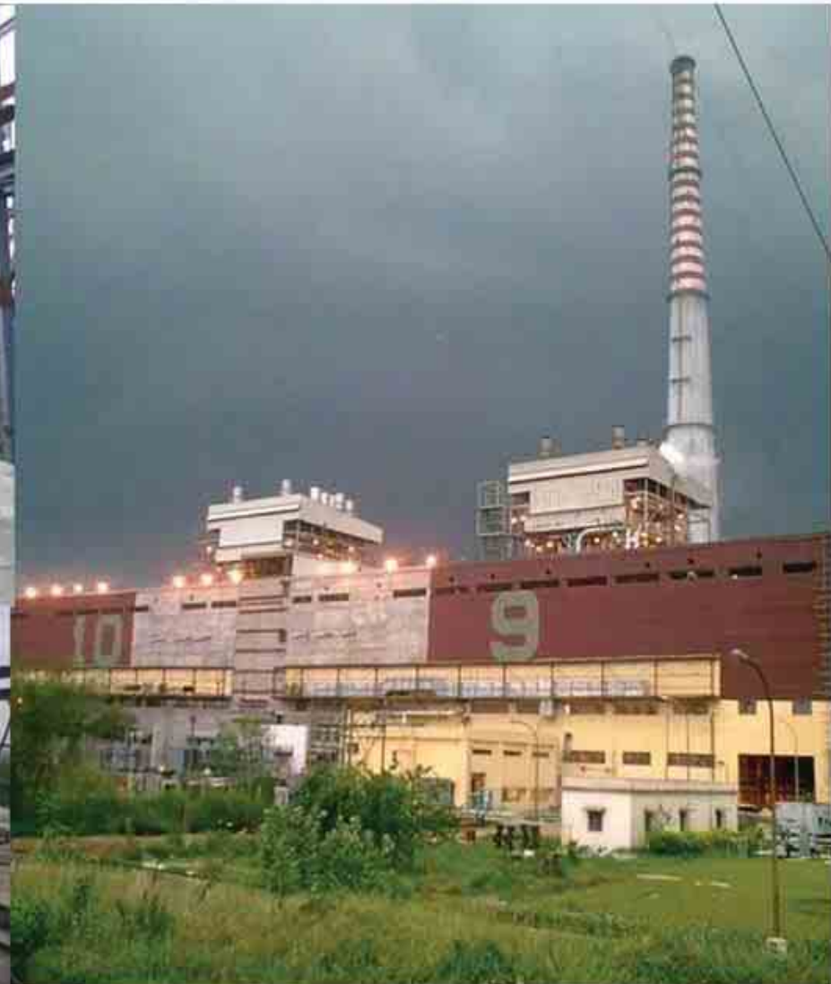
Name of client: BHEL; Work: Site at Angul, Orissa
