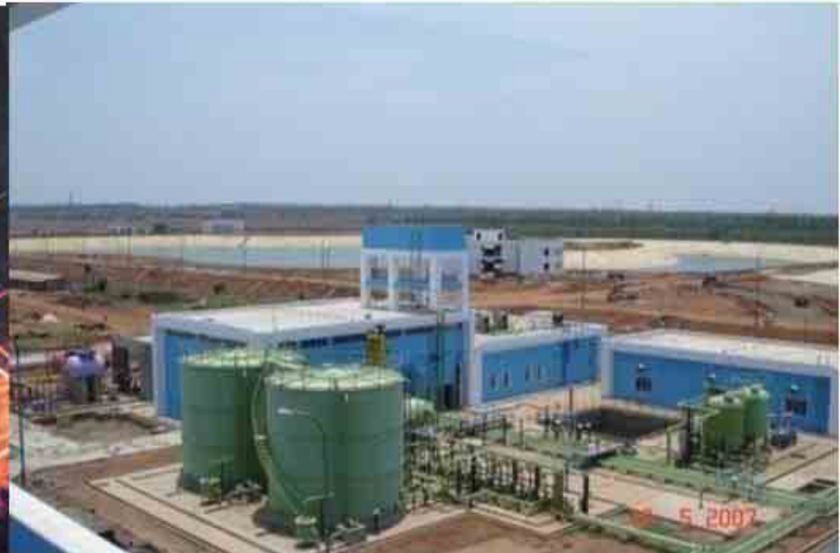
Gautami Power Plant at Peddhapuram, East Godavari Dist, AP
