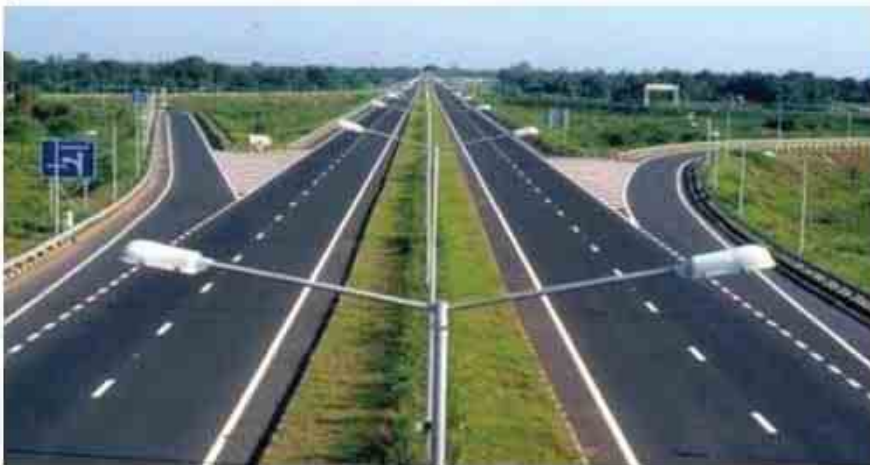
Project: National Express Way No.1(Phase-II of Ahmedabad-Vadodra)
