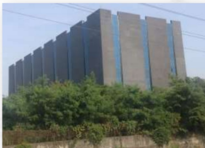
Control's Data Center, Mahape Midc
