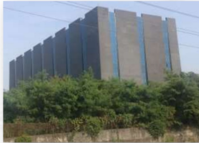
Control's Data Center, Mahape Midc
