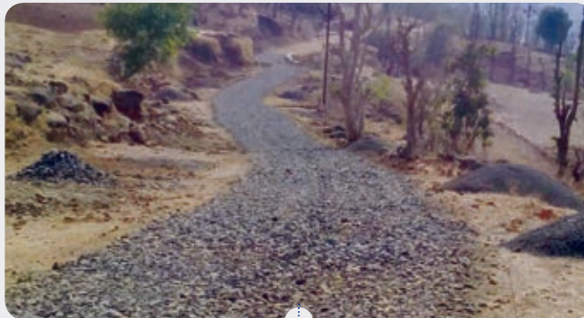
Road connecting Village Biwalpada to Village Dhamani
