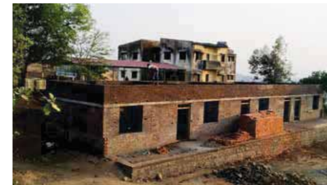
Ashramshala school building under refurbishment
