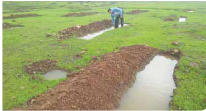
Continuous Contour Trenches at Ase Gram Panchayat after the first showers
