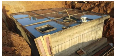
One of the 4 Rainwater Harvesting structures being constructed at Ashramshala
