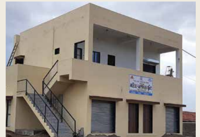
New SHG units being constructed
