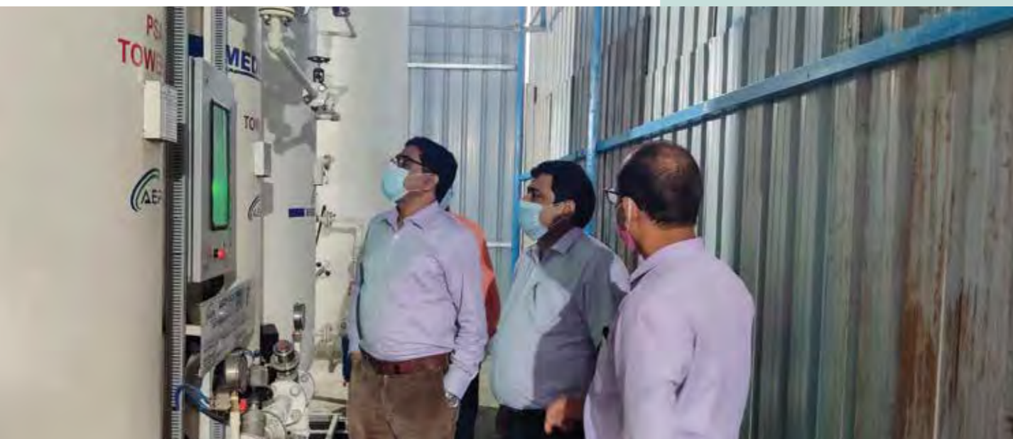
Commissioning and installation of oxygen plant at Mahad
