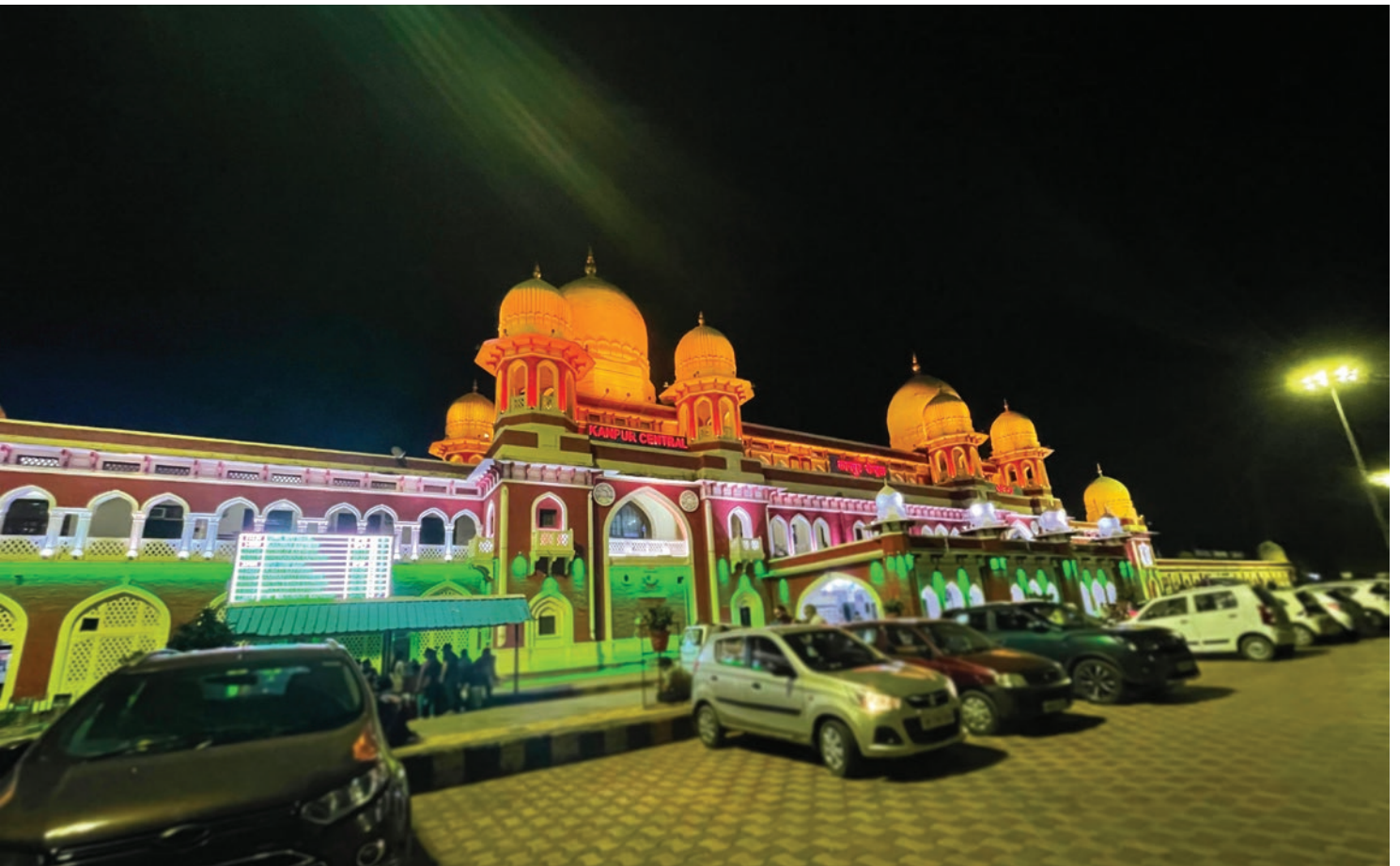
Kanpur Railway Station
