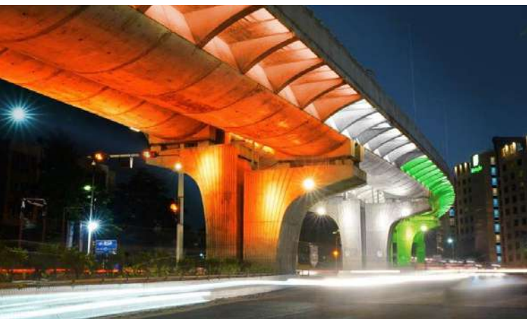
Sodala Bridge, Jaipur
