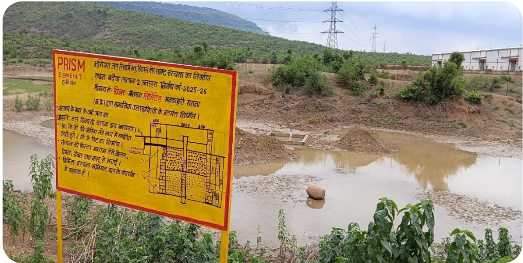
Construction of Water Harvesting Structure at Badhaiya
