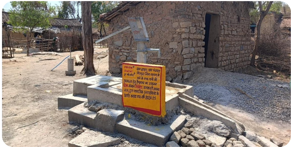
Installation of Hand pump at Jhanjhar Village
