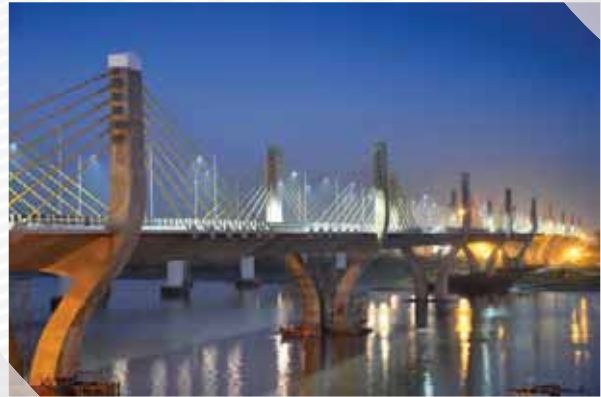
▲ Narmada Bridge Street lighting, Bharuch, Gujarat
