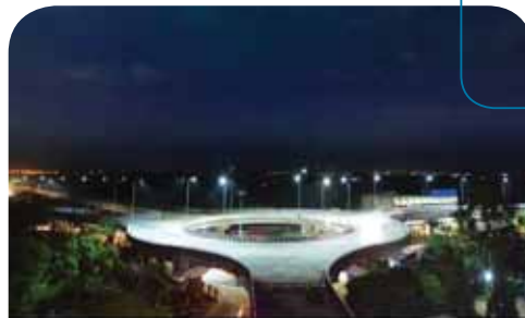
LED Streetlighting at Railway Junction over bridge, Trichy
