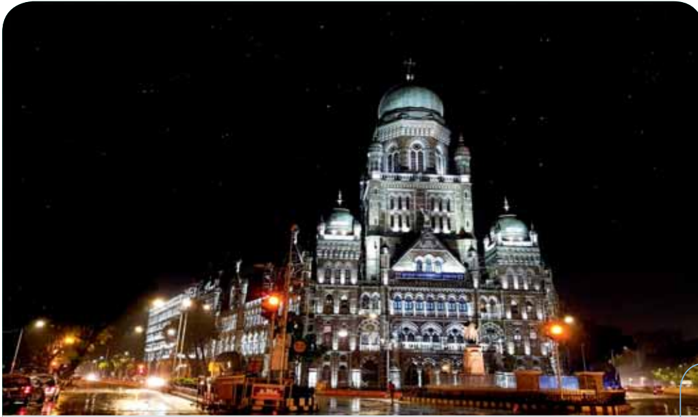
LED Facade lighting at BMC headquarters, Mumbai
