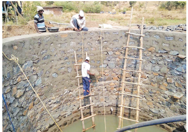
Construction of an open well in Pimpalpada, Maharashtra
