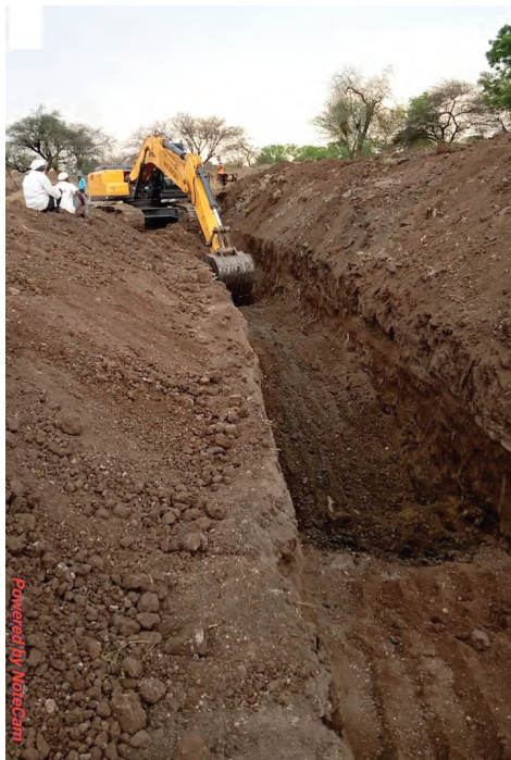
Ongoing nalla deepening work
