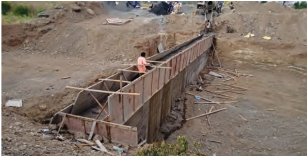
Ongoing work of cement nalla bund
