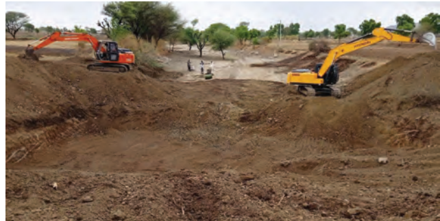
Ongoing work of cement nalla bund
