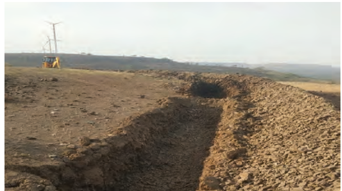
Water Absorption Trench to increase water absorption and reduce soil erosion
