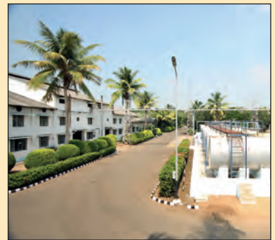
Plant at Ethakota
