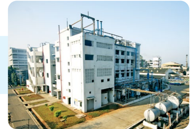
A technical manufacturing plant at Srikakulam in Andhra Pradesh produces technical-grade material for captive consumption as well as for sale.
