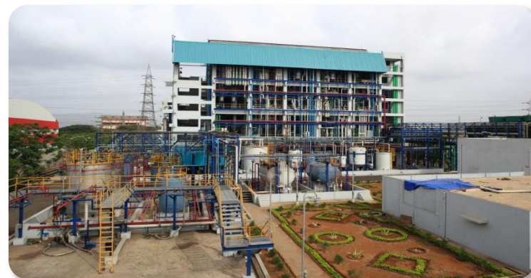
Agro Chemical Facility - Talaja
