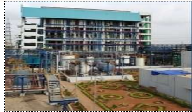
Agro Chemical Facility Taloja
