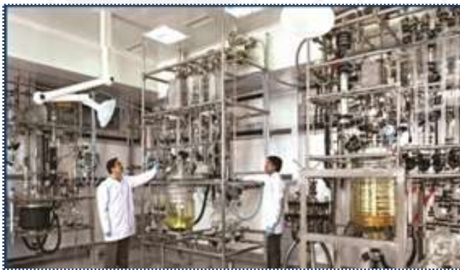
R&D, Contract, cGMP Kilo Lab Pune
