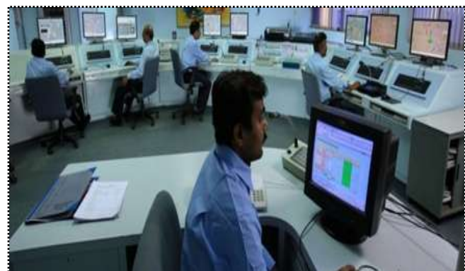
Control Room Taloja
