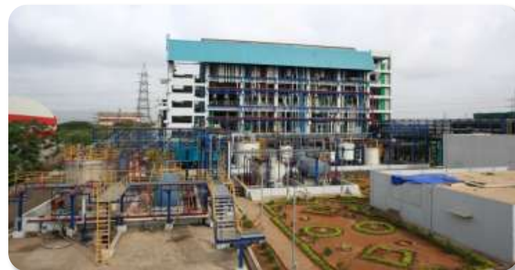
Agro Chemical Facility - Talaja
