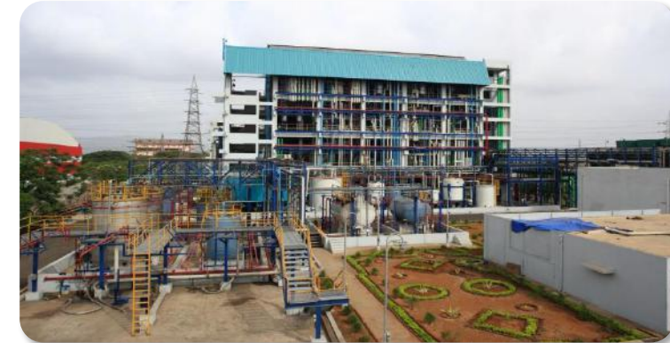
Agro Chemical Facility - Taloja
