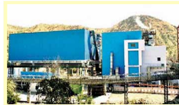
Waste Heat Recovery Power Plant at Jaykaypuram
