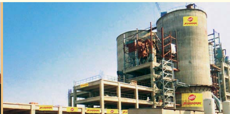
JK Lakshmi Cement's newly commissioned Grinding Unit in Jhajjar, Haryana
