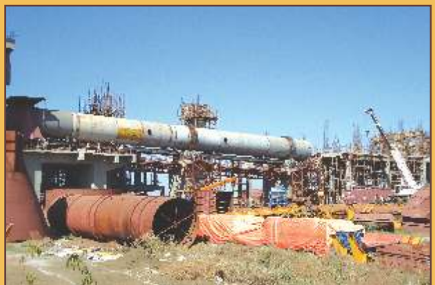
Kiln erection at Durg Plant
