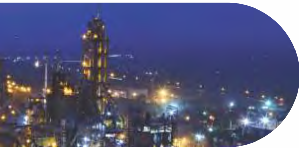
JAYKAYPURAM PLANT - SIROHI
