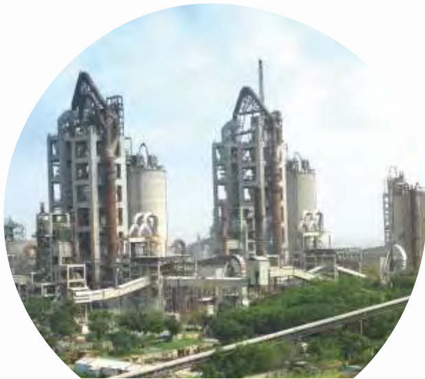
JAYKAYPURAM PLANT - SIROHI
