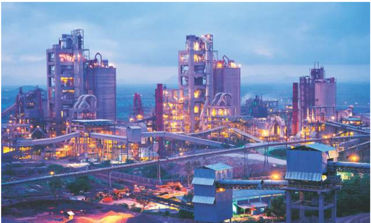
Integrated Cement Unit, Sirahi
