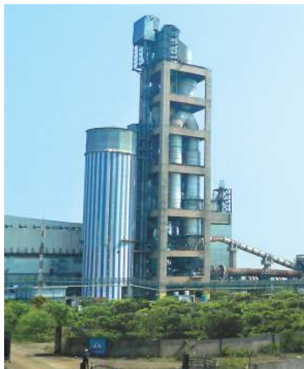
Integrated Cement Unit, Durg
