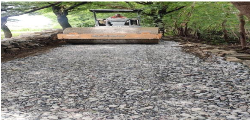
Construction of Gravel road from Bansa to Pipaliya village
