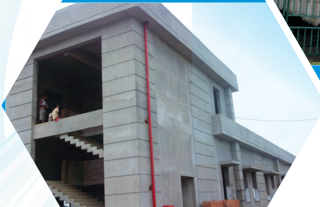
GREATER NOIDA (Factory Under Construction)
