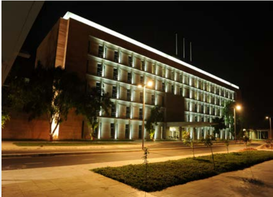
Swarnim Sankul 1 & 2 Construction and interior work
