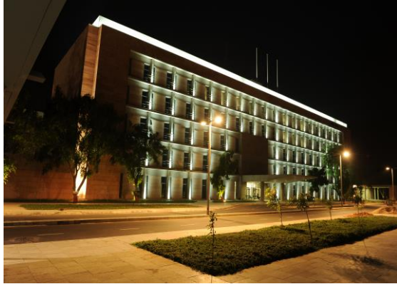
GOVERNMENT OFFICE BUILDING
