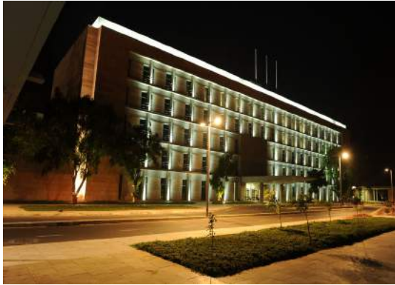
Swarnim Sankul 1 & 2 Construction and interior work
