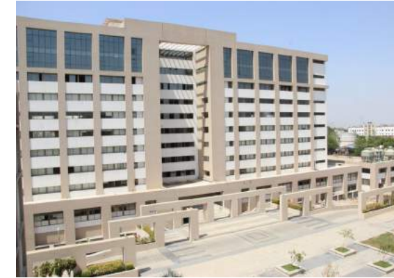
Hospital, Residential Building and Medical College for GCS Medical College, Hospital and Research Centre
