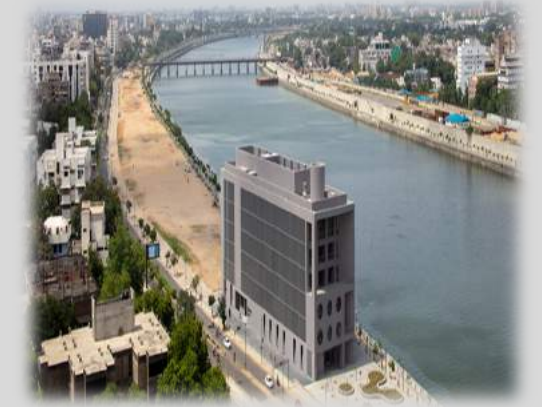
Sabarmati Riverfront Development Co. Ltd. (SRFDCL) Office Building, Ahmedabad
