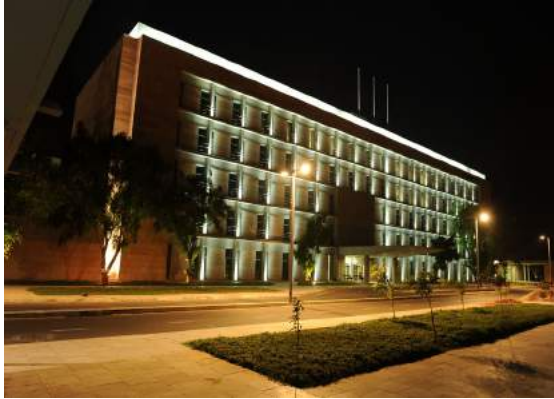
Swarnim Sankul 1 & 2 Construction and interior work
