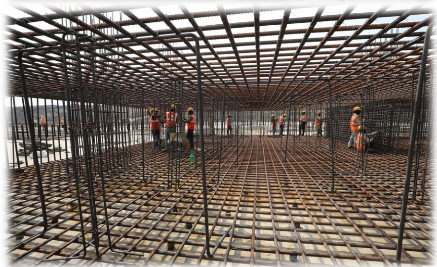
EXCAVATION COMPLETED, FOUNDATION WORK IN PROGRESS
