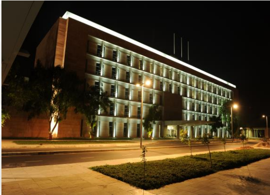
Swarnim Sankul 1 & 2 Construction and interior work
