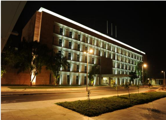
Swarnim Sankul 1 & 2 Construction and interior work
