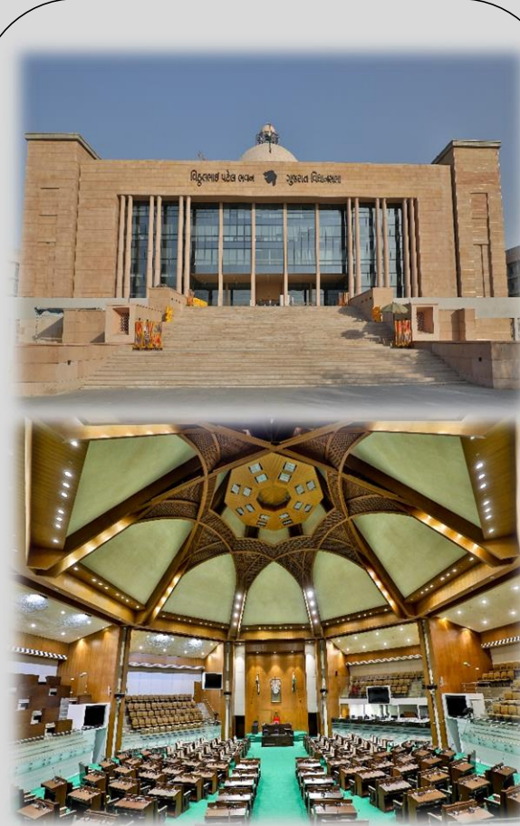
Renovation of Gujarat Vidhansabha, Gandhinagar
