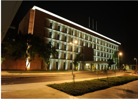
Swarnim Sankul 1 & 2 Construction and interior work
