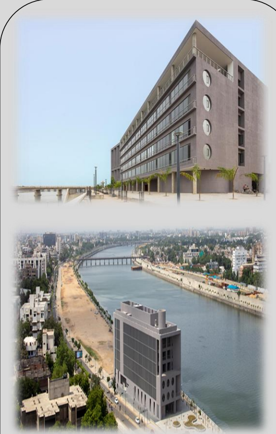
Sabarmati Riverfront Development Co. Ltd. (SRFDCL) Office Building, Ahmedabad
