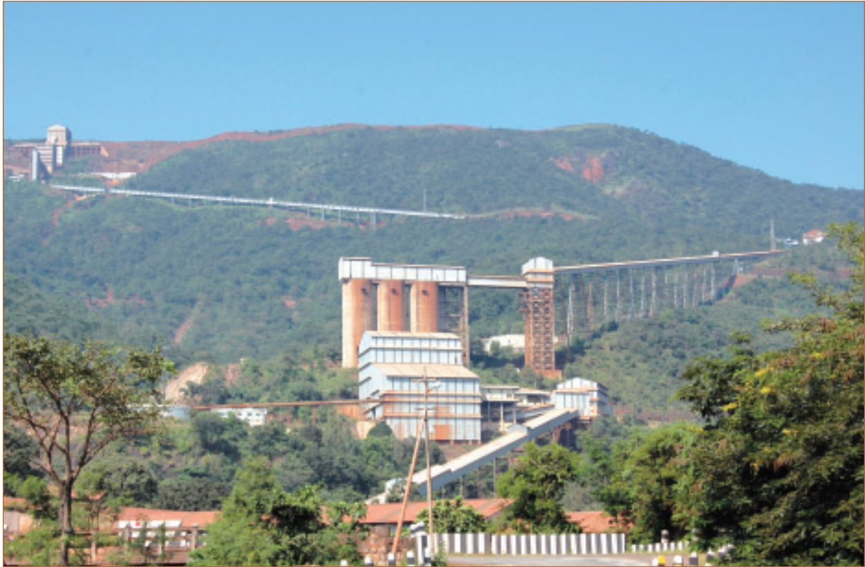
Crushing Plant and Silos of Deposit-10/11A, Bachel Complex, Chhattisgarh
