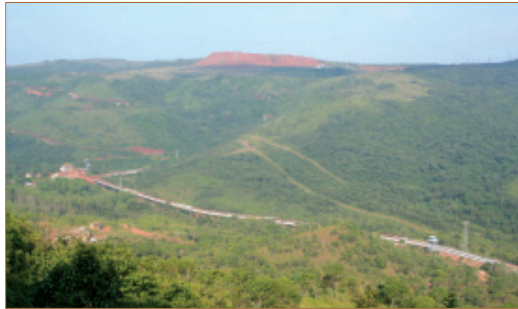
Conveyor System, Bachel Complex, Chhattisgarh
