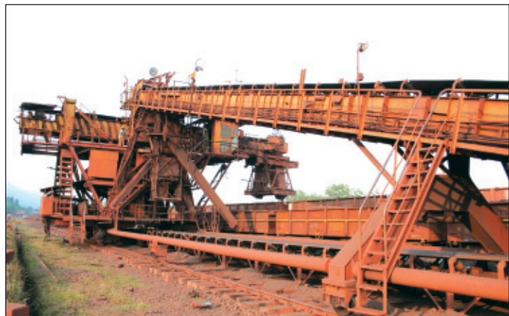
Wagon Loader in Operation
