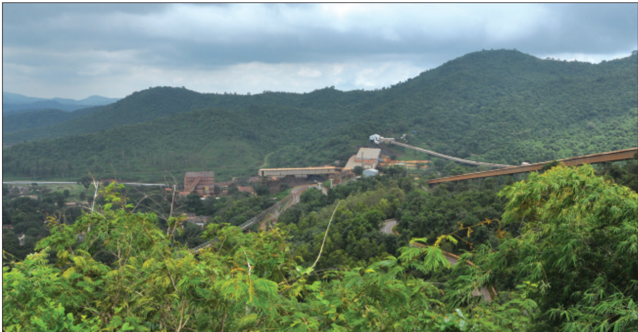
Bailadila Iron Ore Mine, Kirandul Complex
