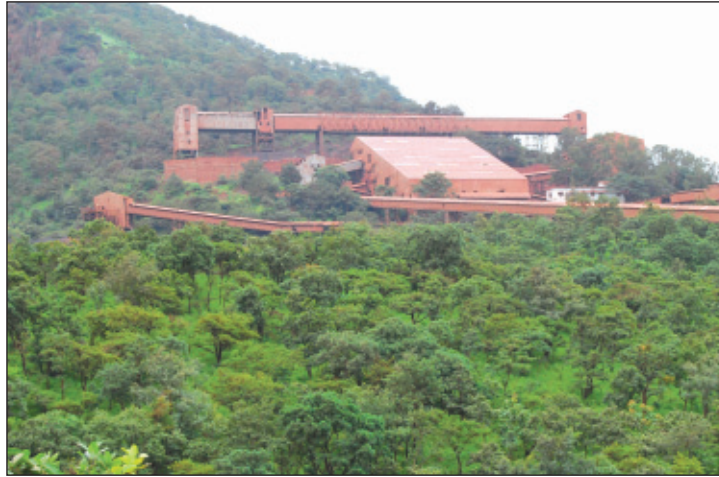
Screening Plant at Donimalai
