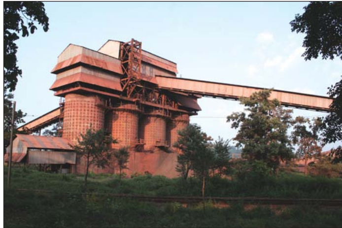
Loading Bunkers at NMDC Mine, Bachel, CG
