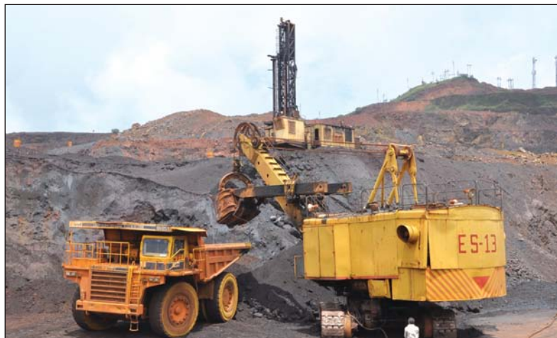
Excavation activity at NMDC Mine
