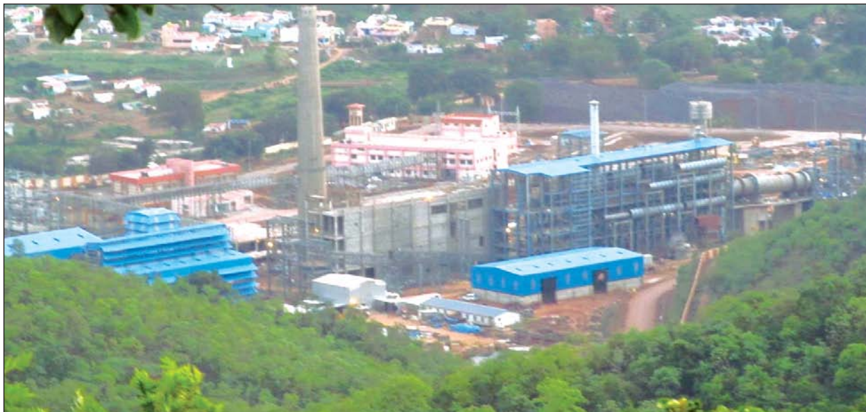
Overview of Pellet Plant, Donimalai under construction
