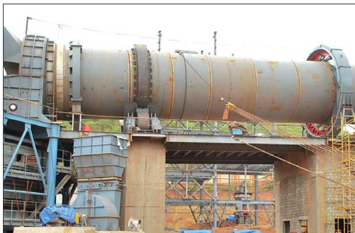
Rotary Kiln at Pellet Plant, Donimalai (under construction)
