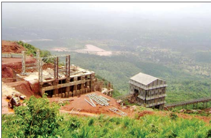
Deposit-11B, Crushing Plant under construction
