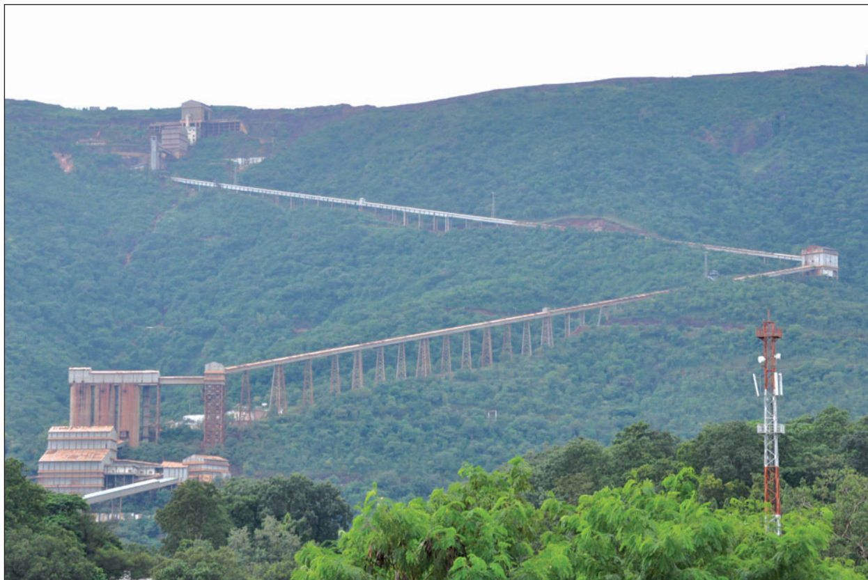
Deposit-10/11A, Bachel Complex, Chhattisgarh
