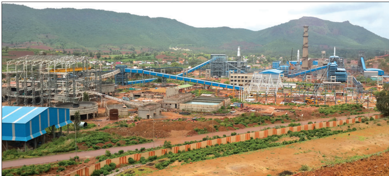
View of Pellet Plant, Donimalai under construction
