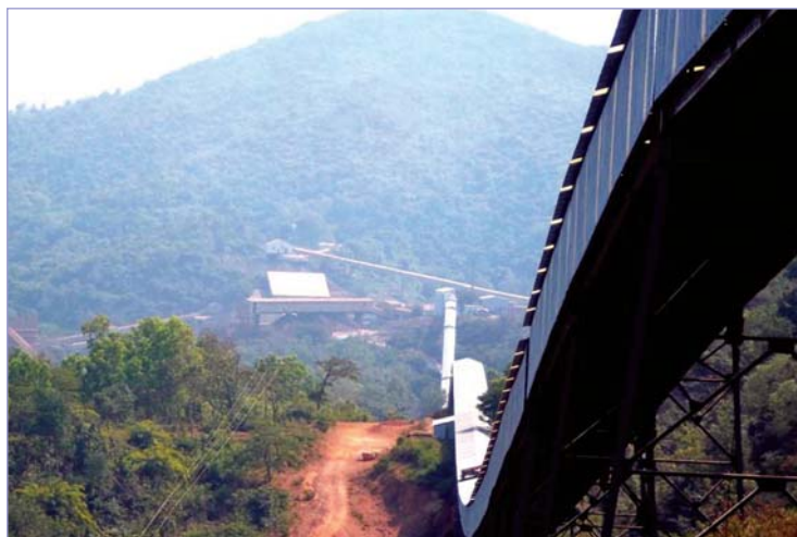
A 3.5 km long conveyor at NMDC's Bailadila Deposit-11B Project
