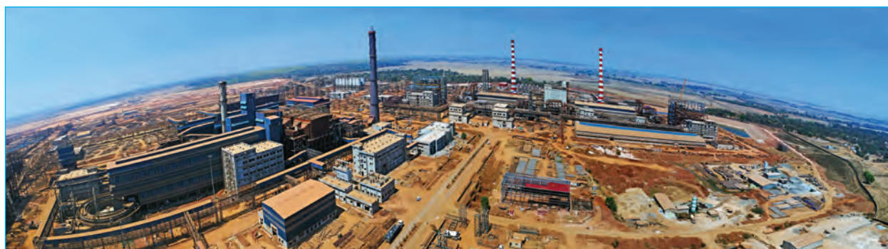
Bird eye view of Steel Plant at NISP, Nagarnar
