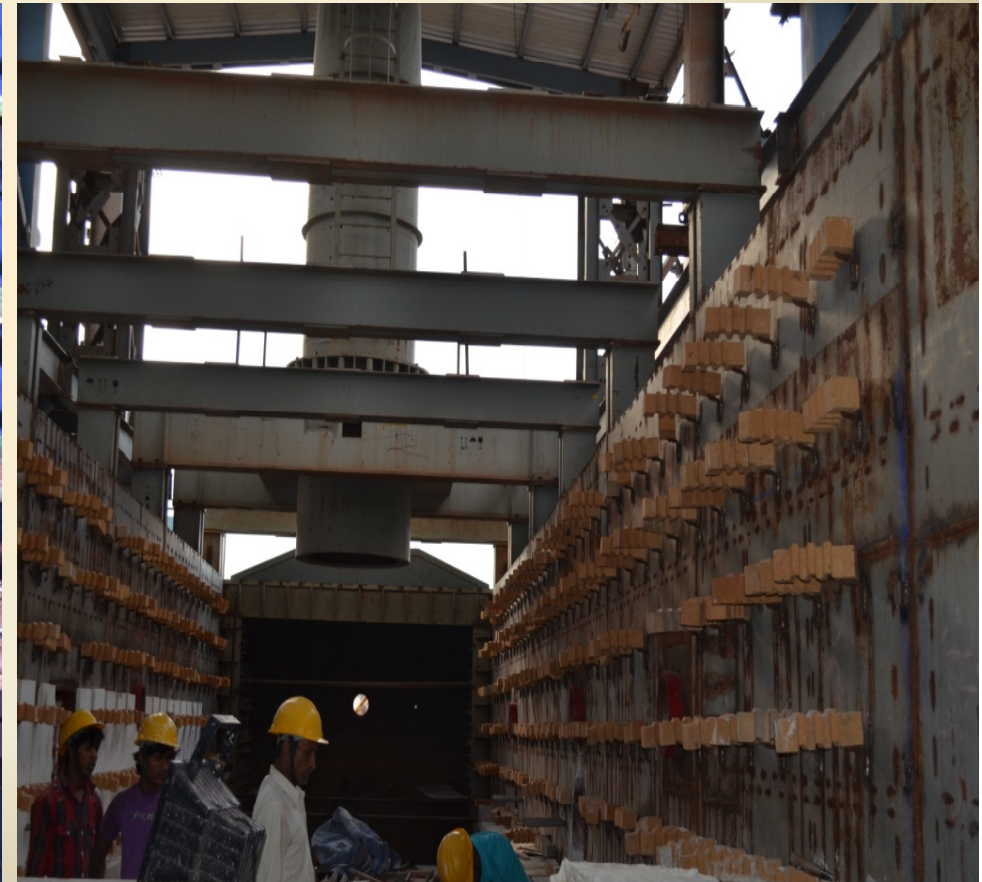
Chain Gate Refractory Erection
