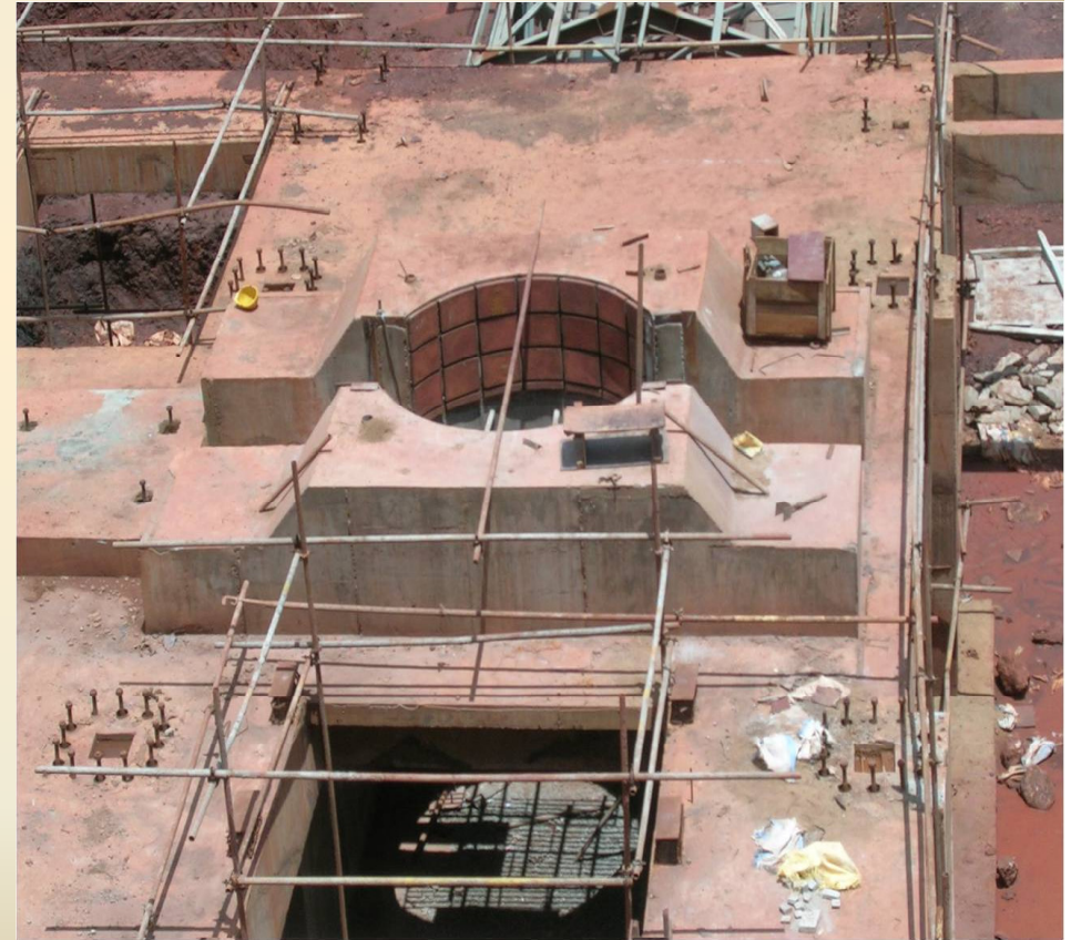
SCH Liner Plat Fixing Work
