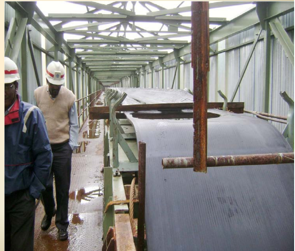
Downhill Conveyor Belt Laying
