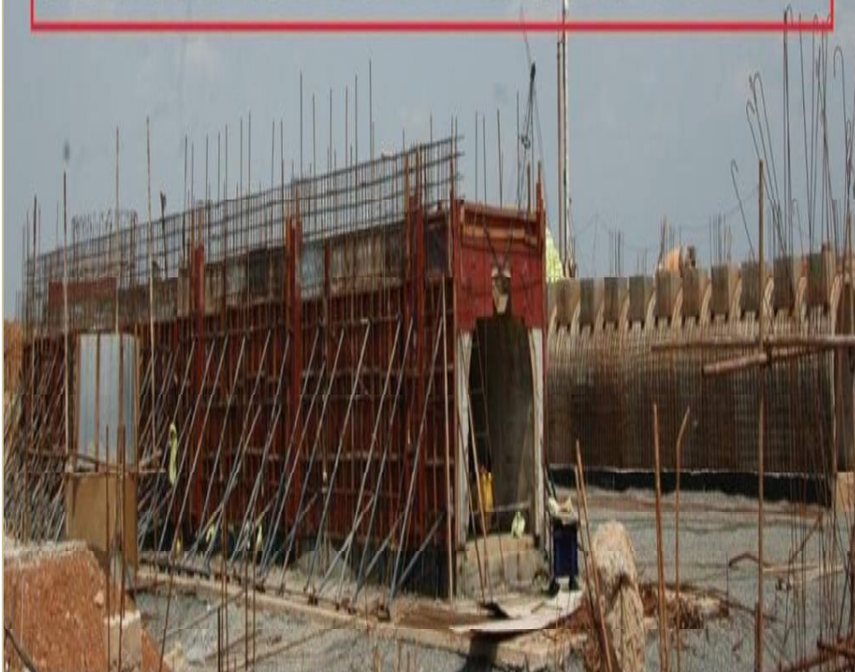
COKE OVEN - SHUTTERING & REINFORCEMENT IN PROGRESS FOR FLUE TUNNEL IN BATTERY2
