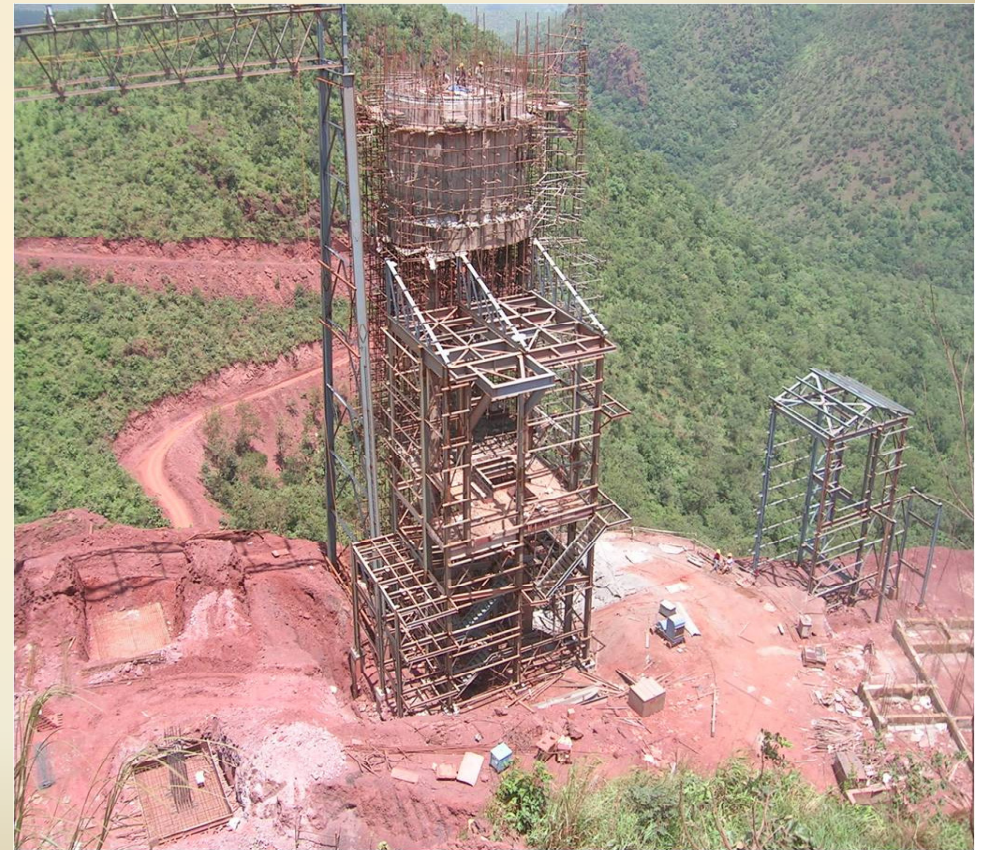
RCC Silo & TH2 TH2A Structural Erection Work
