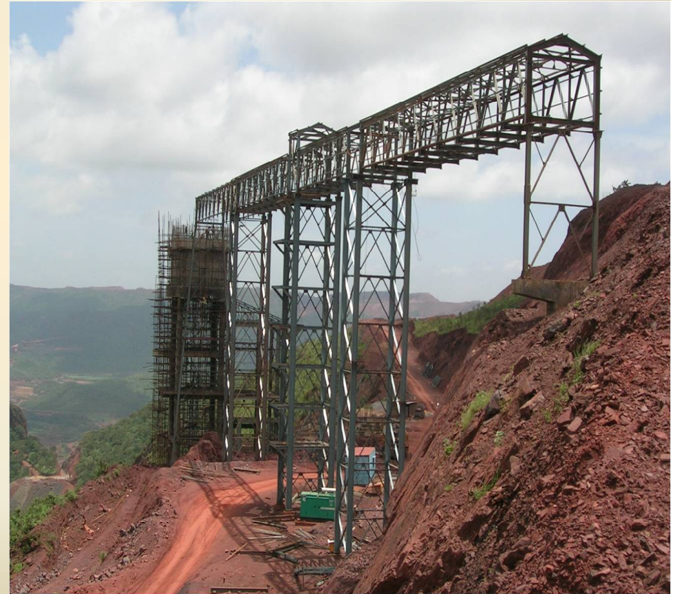
Conveyor 719 Erection Work
