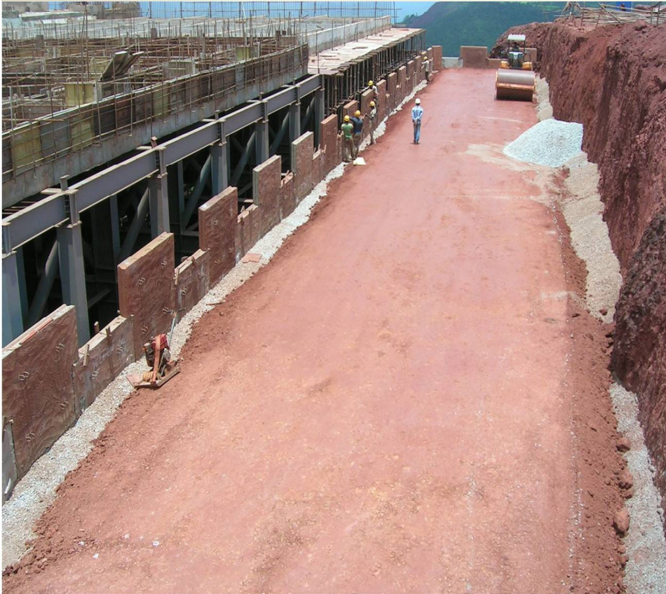
RER Panel Erection and Earth Compaction Work
